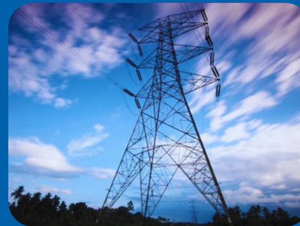
Transmission Tower Projects
