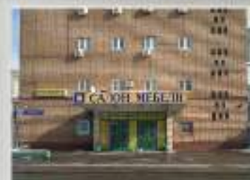
2022-Moskova Ofis/Depo 2022-Moscow Office/Warehouse
