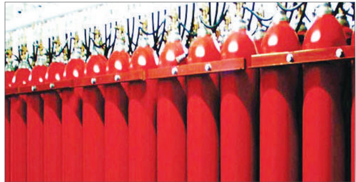
Co2 Fire Suppression Systems
